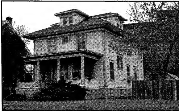
American Foursquare house at 3625 South 24th Street (DO09:0106-011)
